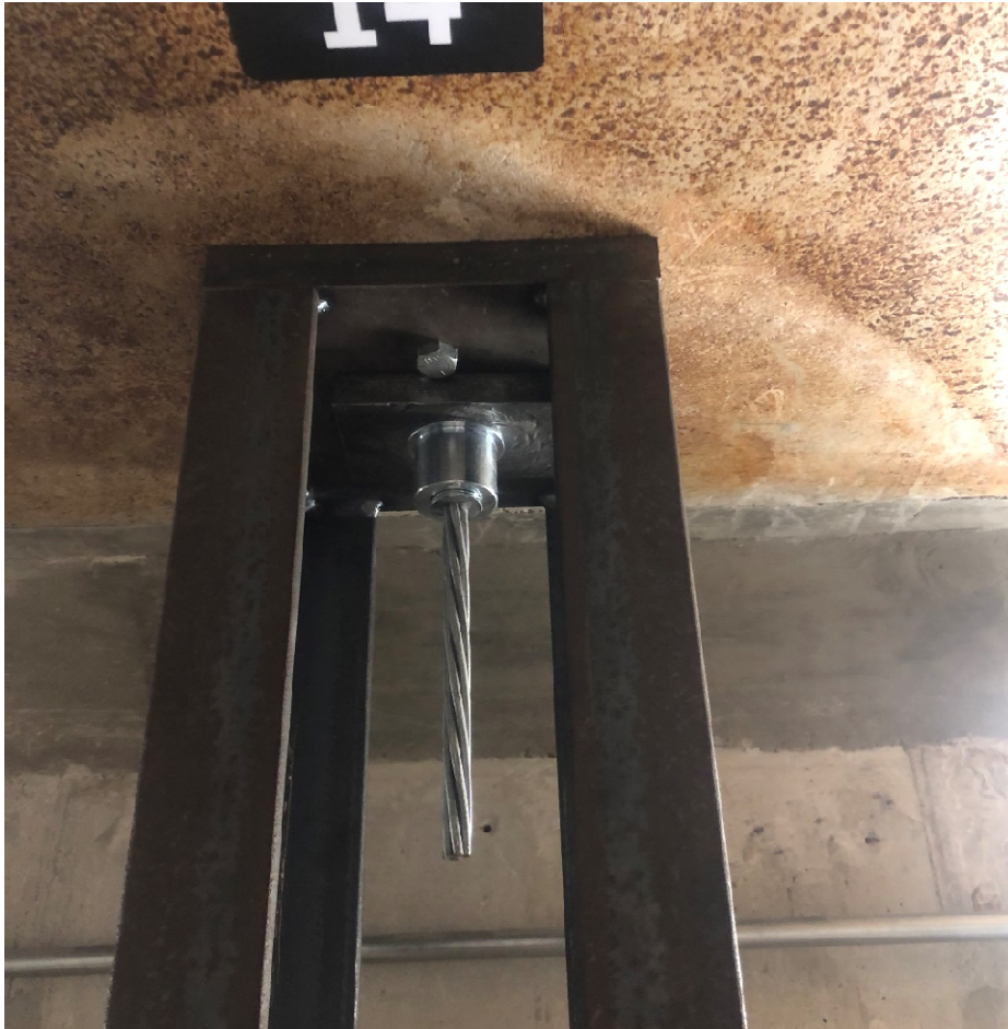
Figure 3. Fatigue anchorage sample bearing on the underside of the structural floor
